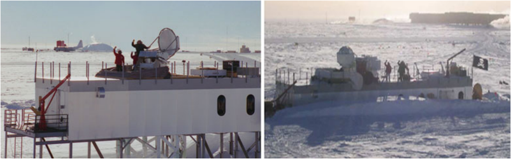
Figure 1. On the left is a picture taken of AST/RO in the late 1990's, a few years after its construction. For contrast, another picture of AST/RO taken in late 2005 during decommissioning is shown on the right. You can clearly see how the snow level has risen around the building over the course of the decade due to drifting in the Dark Sector at the South Pole.
