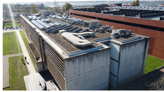
Figure 2: Geosciences department of Aveiro's University - South façade
