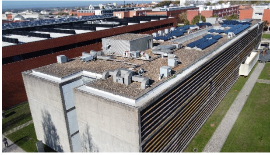
Figure 1: Geosciences department of Aveiro's University - South façade
