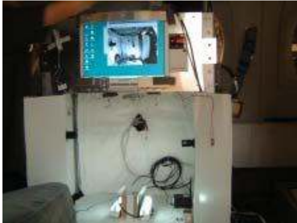
Figure 7.38 Control panel/PC (Control panel toward the passenger's seat and shielding the monitor from outside light with a gatefold cover)
