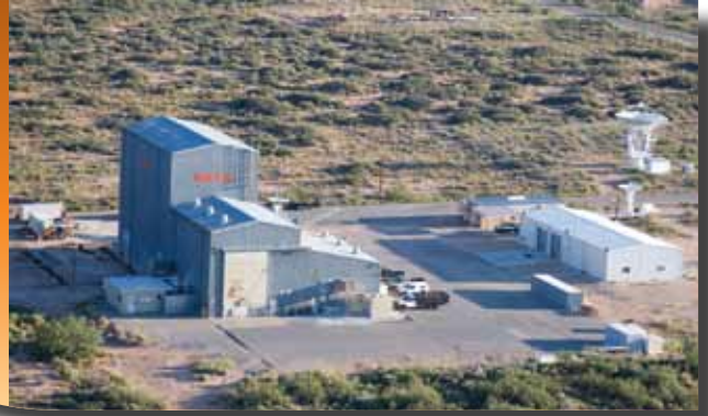
VAB construction at WSMR.
