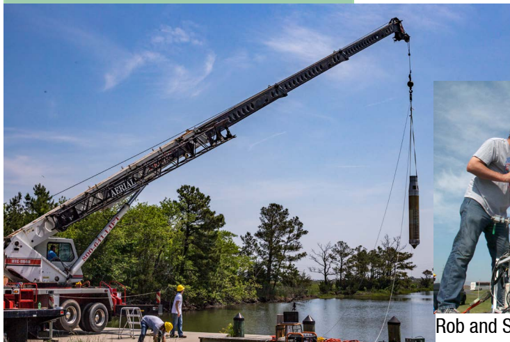
Water recovery system ready for drop.
