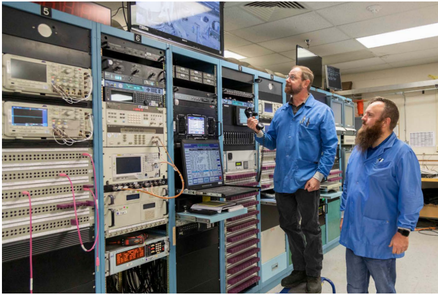
Ground station three upgrades in progress.
