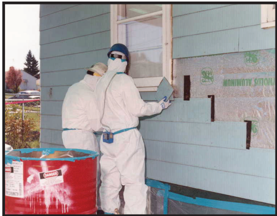
Removing siding
