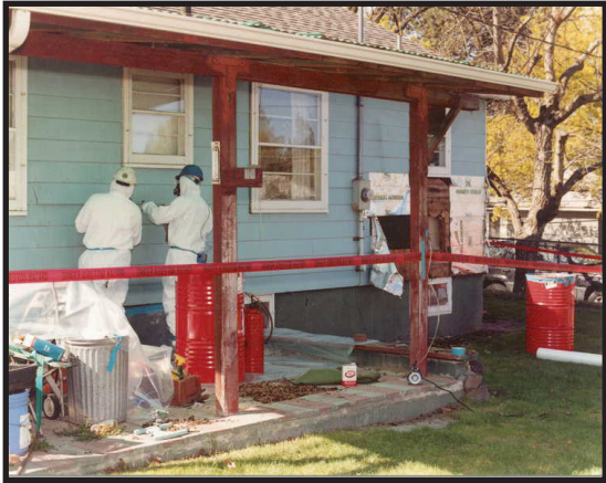
Prying to expose nail heads
