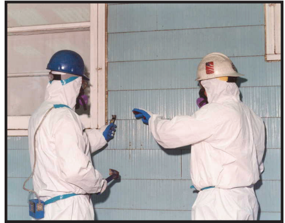
Pulling out nails
