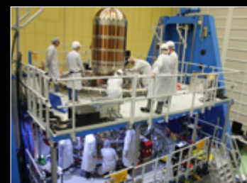
Fuel tank installation
