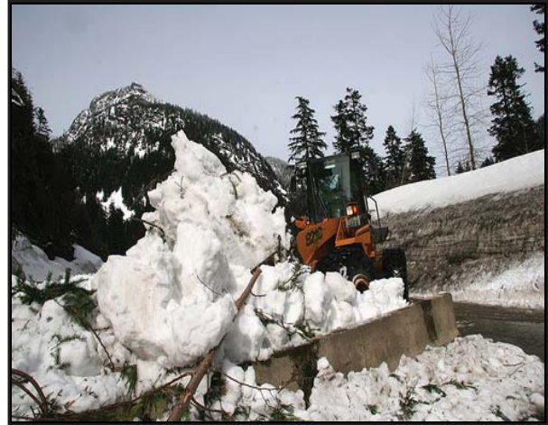
Crews working to clear an avalanche on I-90
