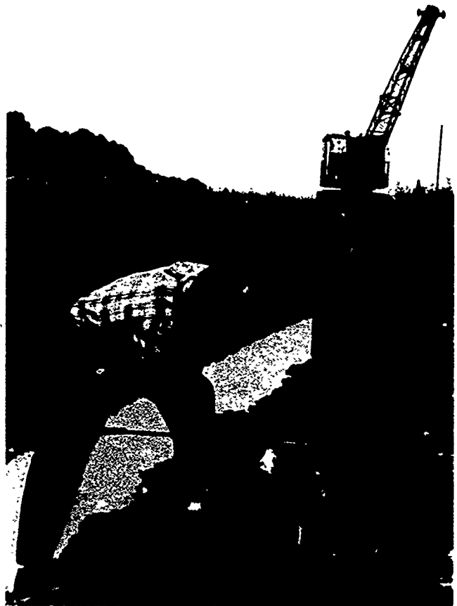
Figure 2-10—This group drainage ditch, formed through dragline construction, replaces an inadequate and obstructed 24-inch tile outlet. The new ditch serves 900 acres on seven farms near Gniffin, Ohio.
