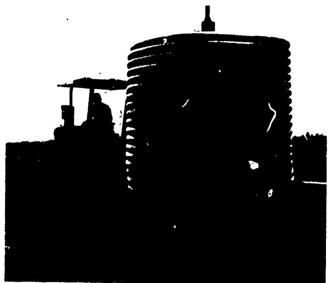
Figure 3-5—(left) A farmer tows a trailer that uncoils 3,000-foot maxi-coils. A wagon stands ready to install 250-foot coils of 4-inch diameter plastic drainage tubing.
