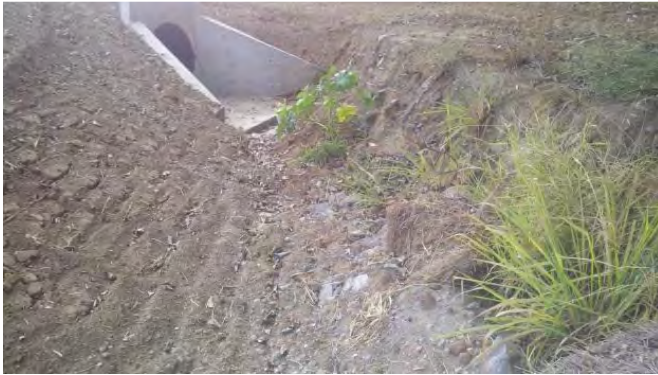
Figure 3.6 Outlet of the storm culvert
