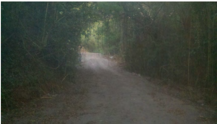
Figure 2.3 A finished section of the road built with AES coal ash.
