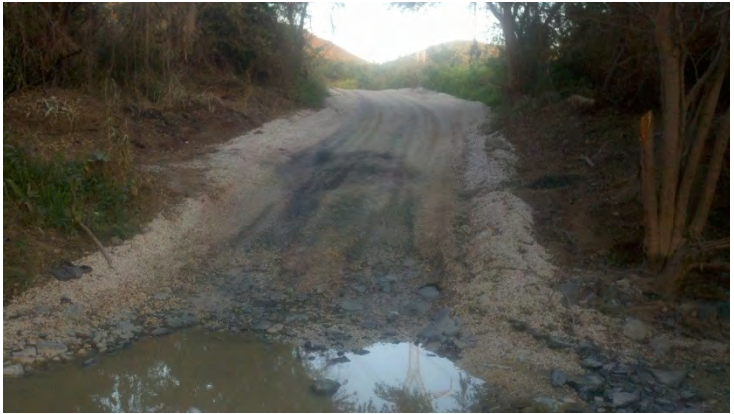
Figure 1.3 AES coal ash poured across the Seco River and washed out by the river
