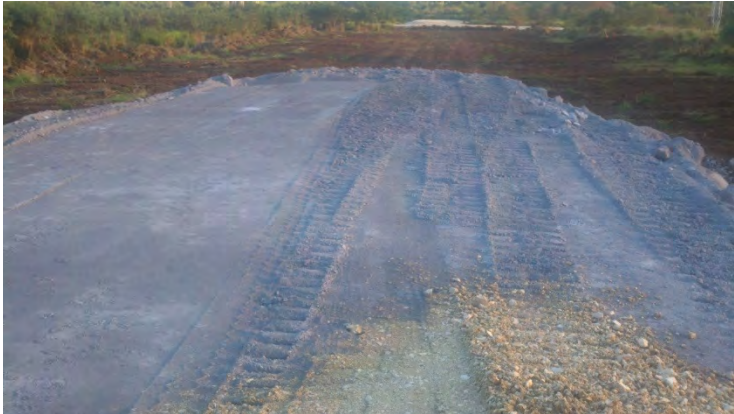
Figure 1.2 New section of the road built with AES coal ash.
