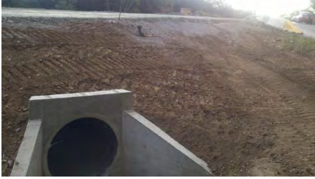
Figure 3.5 View of the storm culvert
