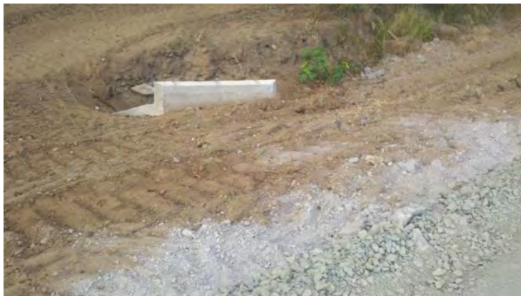
Figure 3.4 AES coal ash residues drain into the stormwater system
