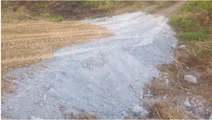
Figure 1.1 Portion of the road showing how the AES coal ash is covered with a thin layer of dirt.
