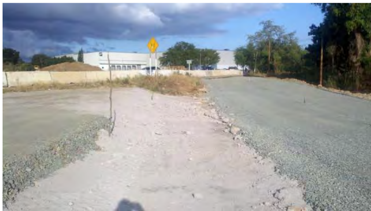
Figure 3.3 A layer of concrete dust poured over the AES coal ash
