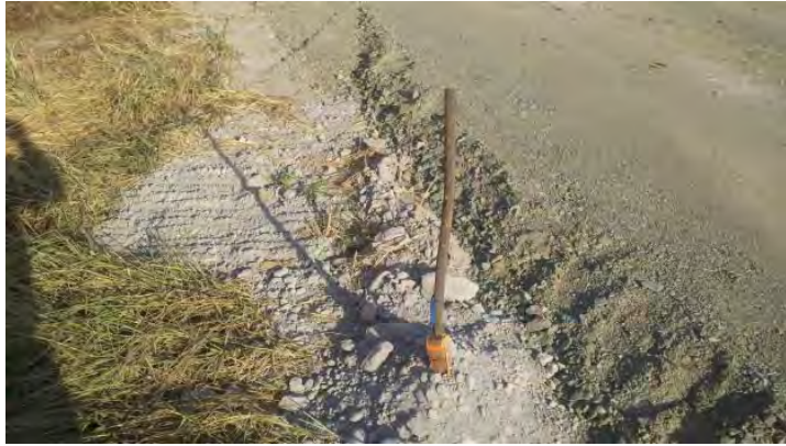
Figure 3.2 AES coal ash used as base fill.
