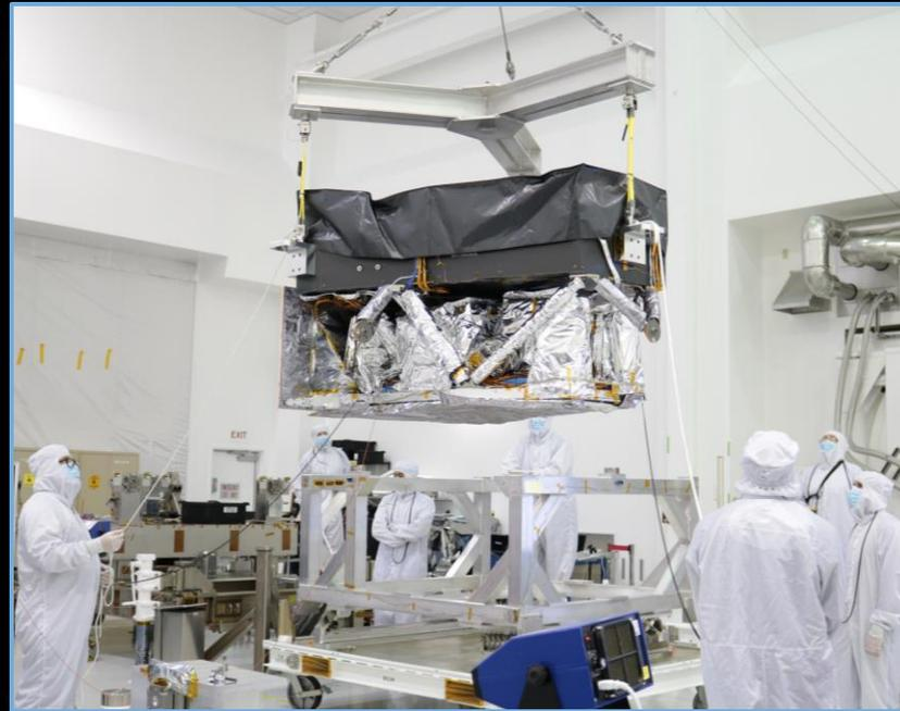
*Post Full Functional Test lift onto shipping container which will be used to transport CGI to electromagnetic-testing facility*
