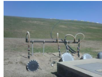
Riser Gas Tie-In from Active Cell
