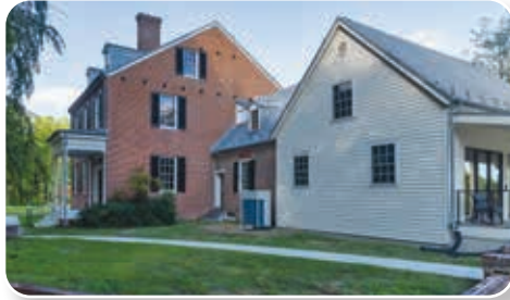
Woodlawn House, with its three primary sections: the 1970s wing in white, the 1735 kitchen in the center, and the three-story 1841 wing. (Credit: Christine Dunham/SERC)
