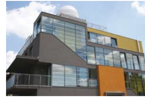
Astronomical pavilion – the new building of the Institute in Prague.
