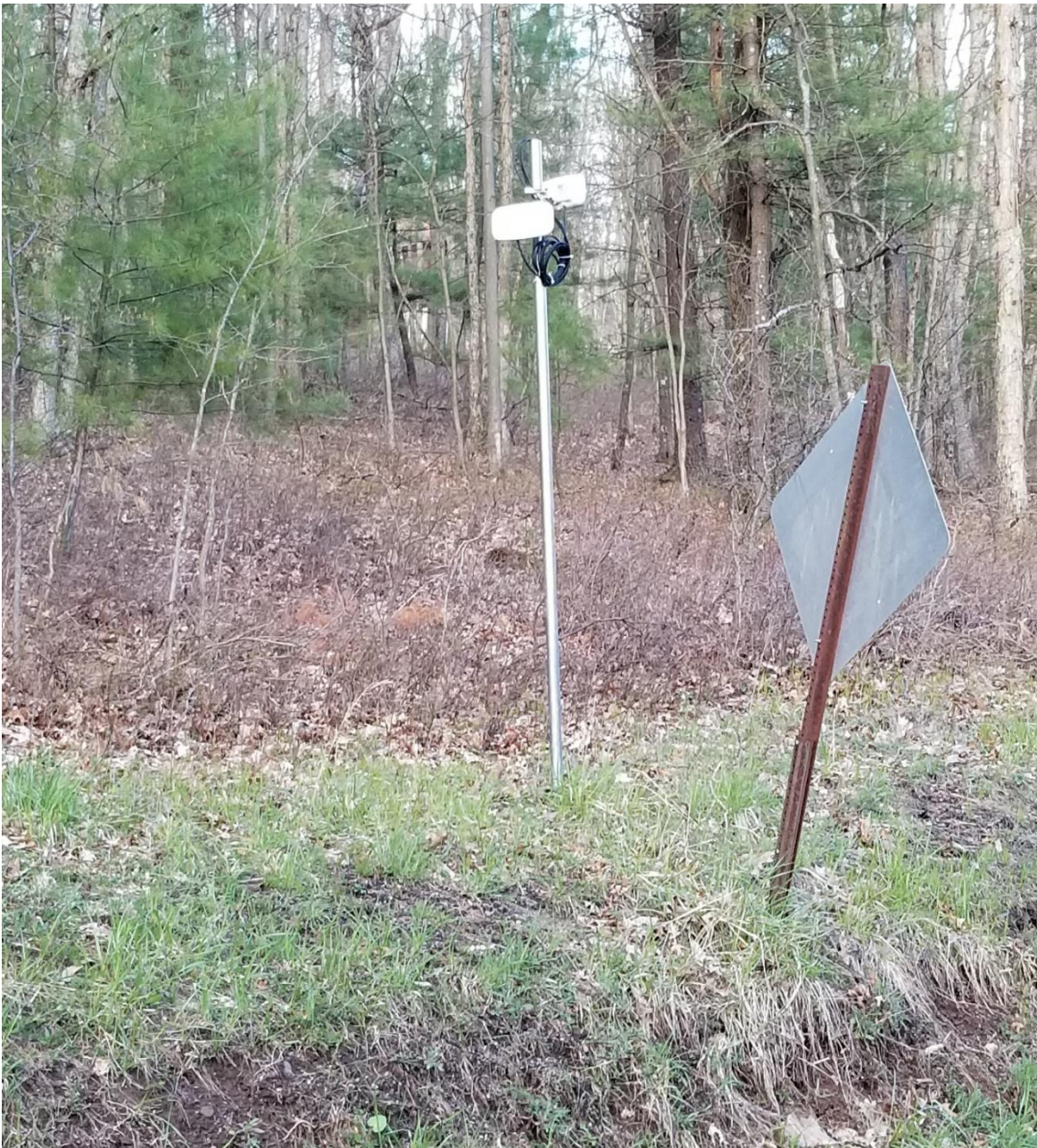
Figure 13: Ad-hoc antenna installed by a WISP
