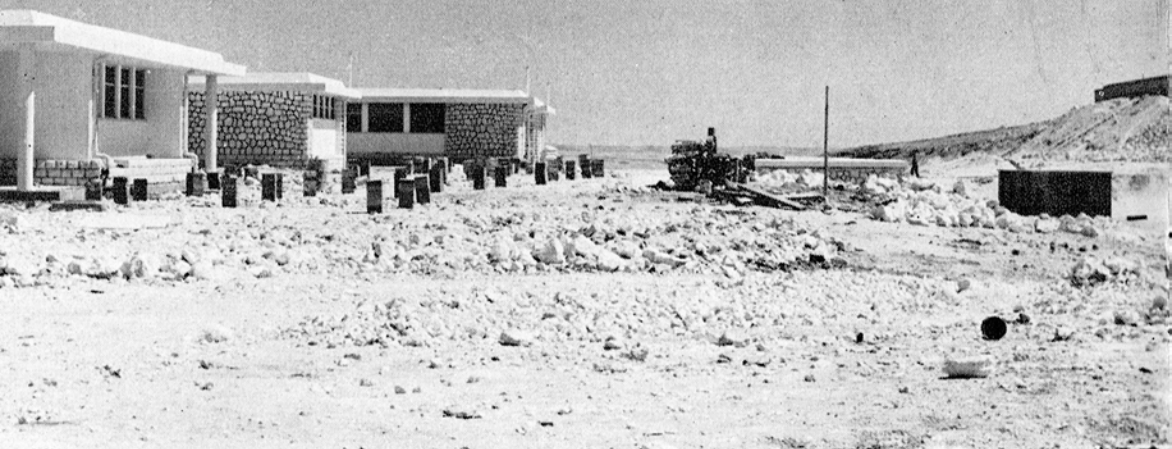
This recent picture shows work presently under way at the
