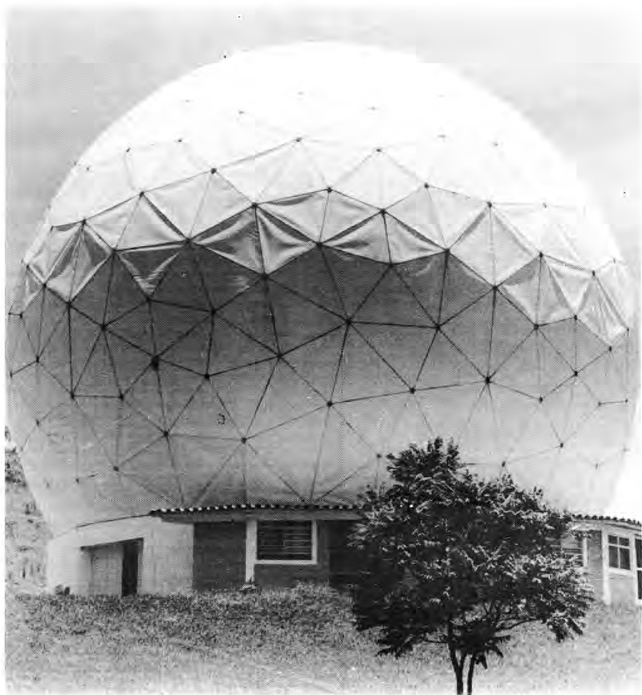
The 13.7-m radome-enclosed telescope was built in 1971 at Itapetinga Radio Observatory (near São Paulo) and is used extensively for VLBI, solar physics, and other radio astronomy programs.
