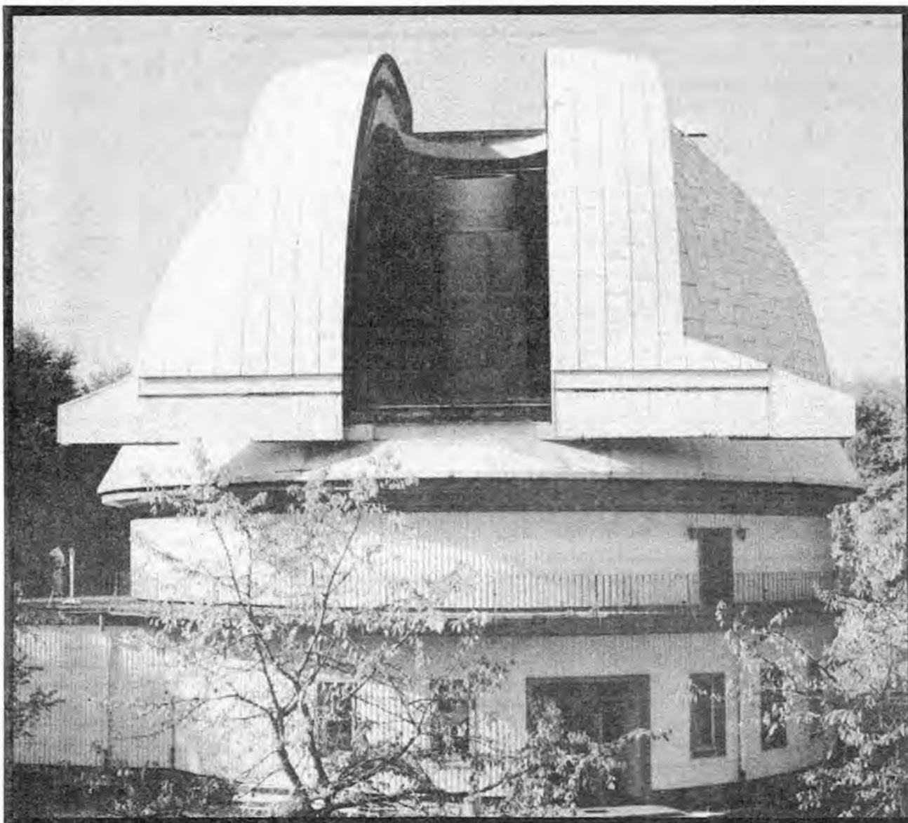
Dome of the Karl Schwarzschild Observatory at Tautenburg. It shelters a 2-meter telescope which, uniquely in the world, can also function as a 52" Schmidt telescope.
