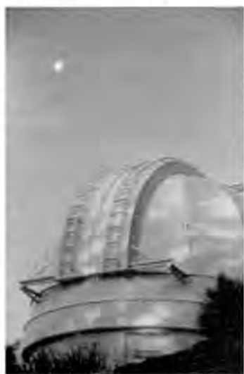
The dome of the 24-inch TiE telescope on Mount Wilson, California.
