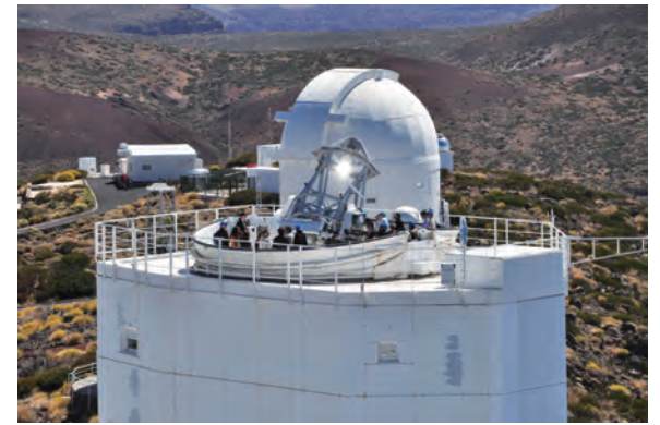
Fig. 2: Inauguration of the 1.5-meter GREGOR solar telescope at Observatorio del Teide, Tenerife, Spain on May 21, 2012. The bright spot in the center of the picture is a reflection from the heat-stop rejecting all sunlight except for a small field-of-view of about 150 seconds of arc in diameter.
