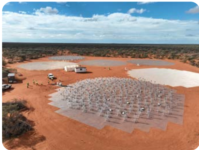
Bird's eye view of Low-Station S8 with two completed stations.
