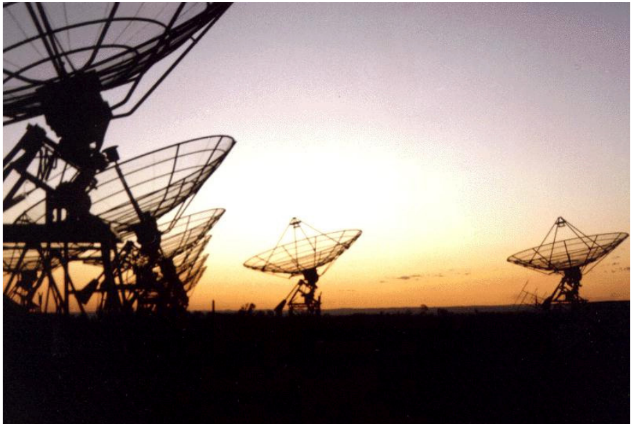
Figure 1: Part of the 32-element Chris Cross solar grating array near Sydney, used by the current President of C3 back in the 1960s. Credit: John Leahy.
