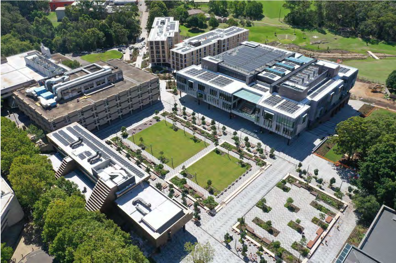
Image 2: MUCCP Central Courtyard Precinct
