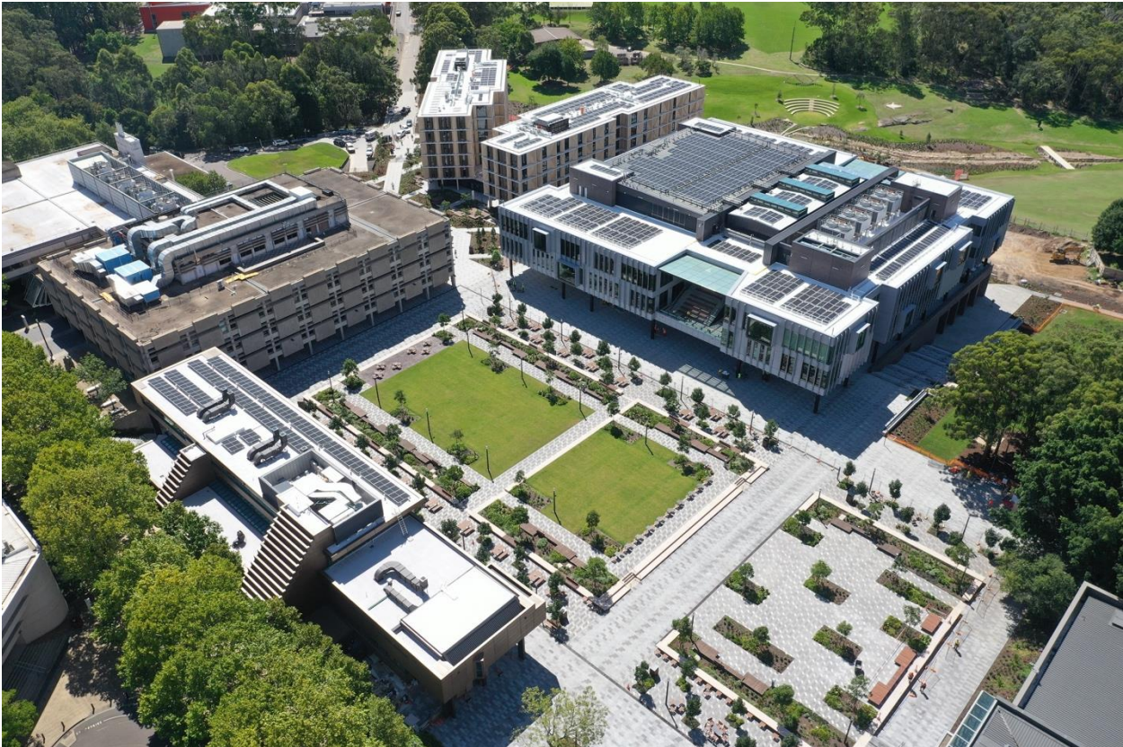
Image 2: MUCCP Central Courtyard Precinct
