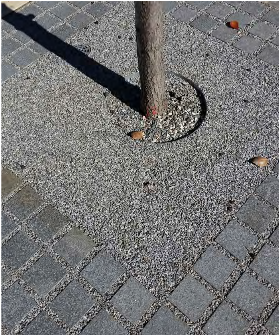
Figure 14 The metal surround should be removed well before the trunk outgrows the circumference.
