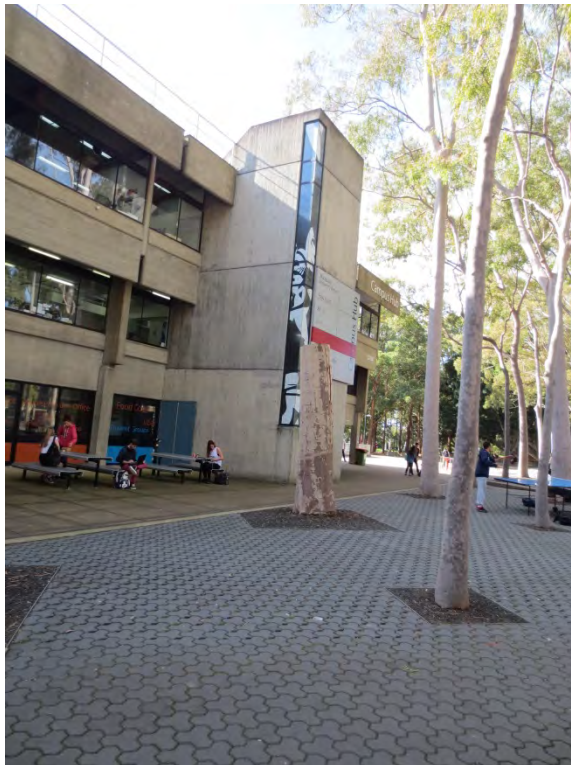
Figure 32 Dead Lemon Scented Gum should be replaced.
