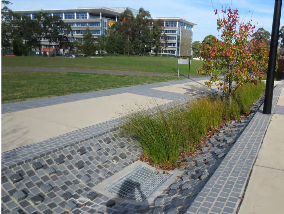
Figure 22 A partially planted drainage swale in the Cochlear Forecourt.
