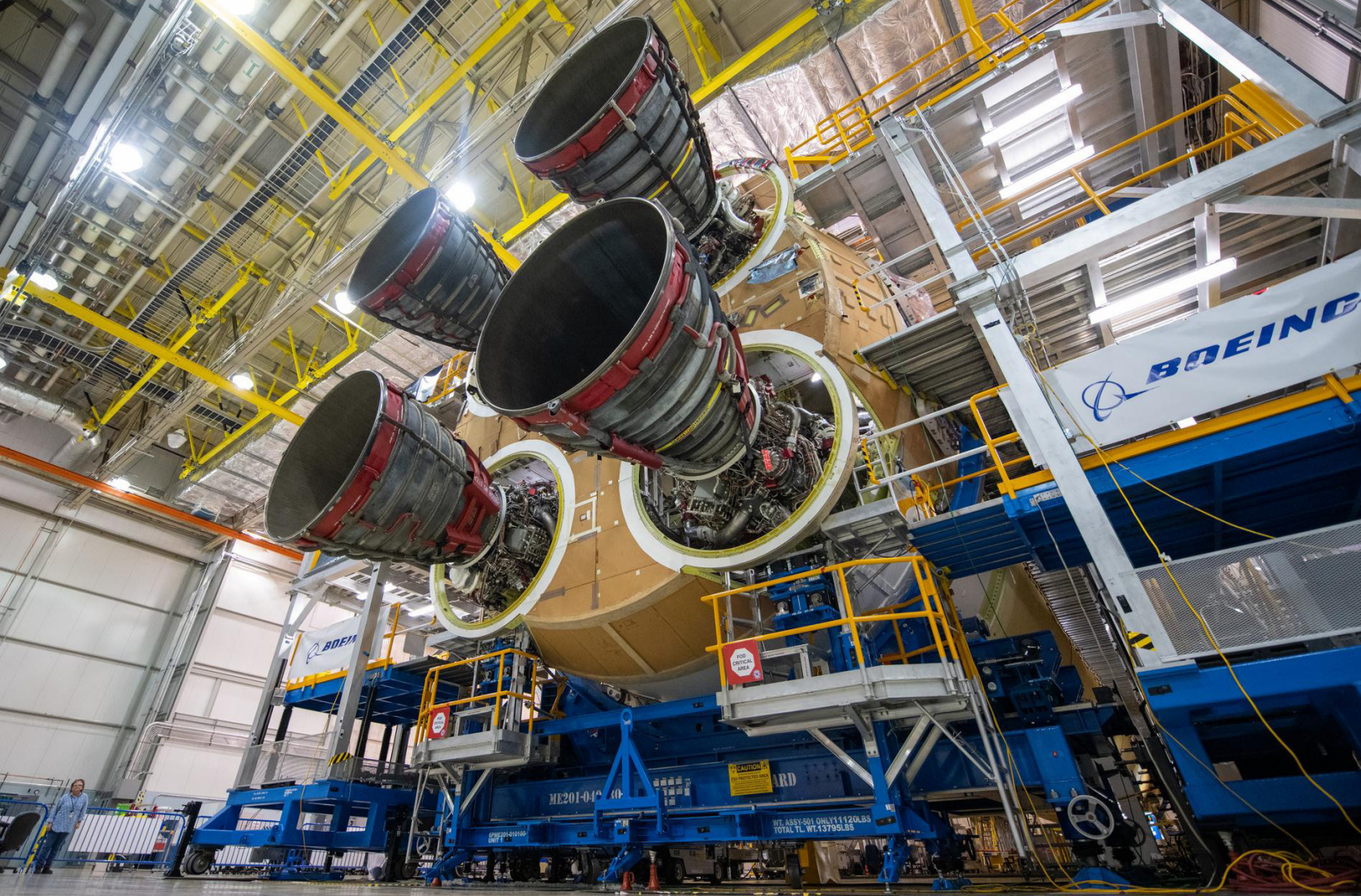
Completed Space Launch System (SLS) Core Stage at Michoud Assembly Facility (MAF) Credit: NASA/Jude Guidry
