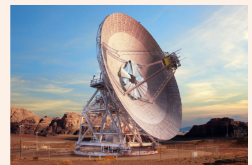
Artist's concept of Deep Space Station 23, a new antenna dish being constructed at the Goldstone, California, DSN complex. (NASA)
