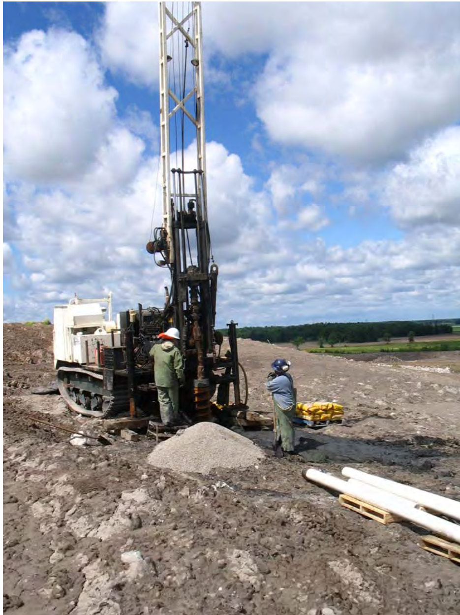
Photo 3: Vertical Landfill Gas Extraction Well Drilling and Installation
