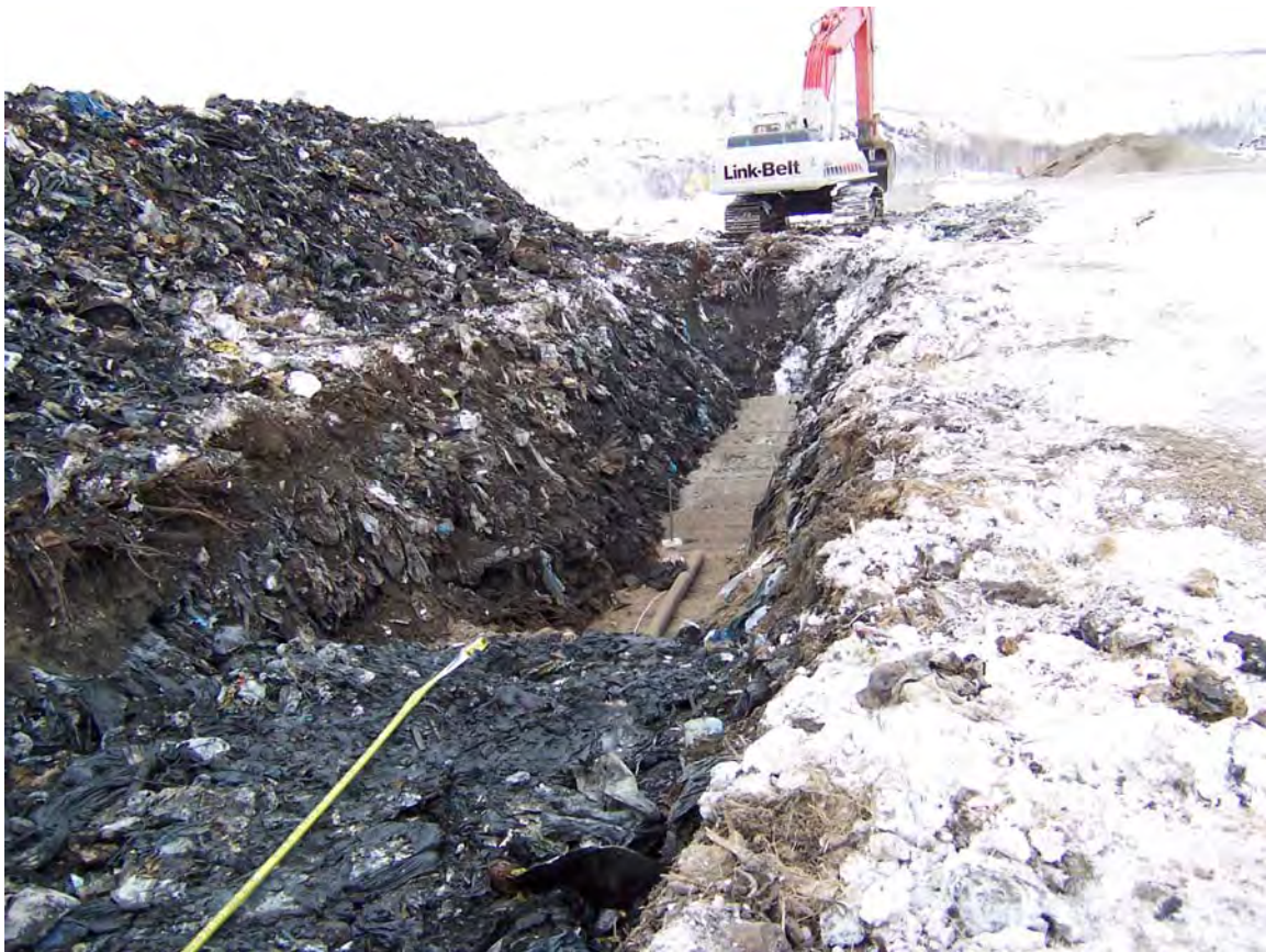
Photo 2: Horizontal Landfill Gas Collection Trench Installation
