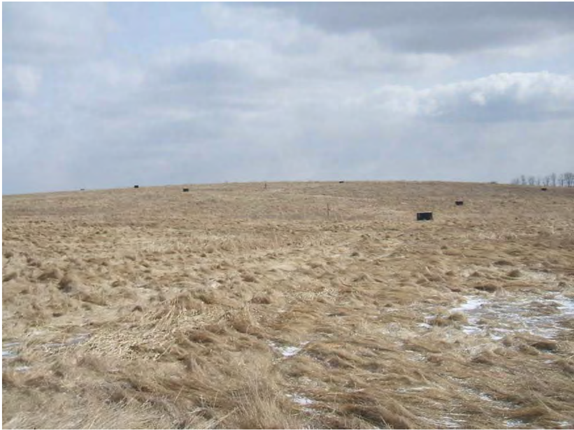
Photo 6: Vertical Landfill Gas Extraction Wells in Above-Ground Chambers
